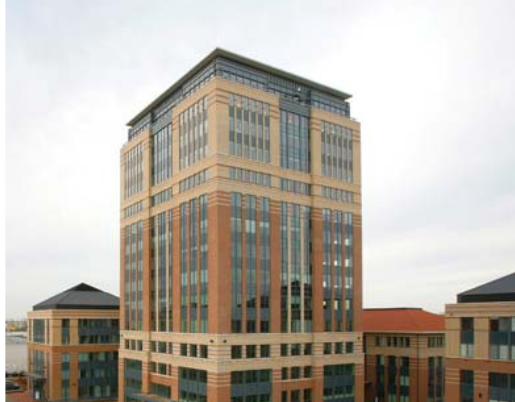
Mechelen Campus Tower Mechelen
