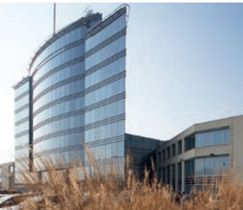
□ Mechelen Business Tower - Malines
