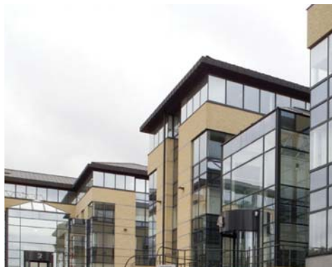
11. INTER ACCESS PARK
