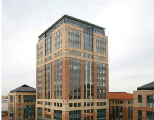
Mechelen Campus Tower Malines
