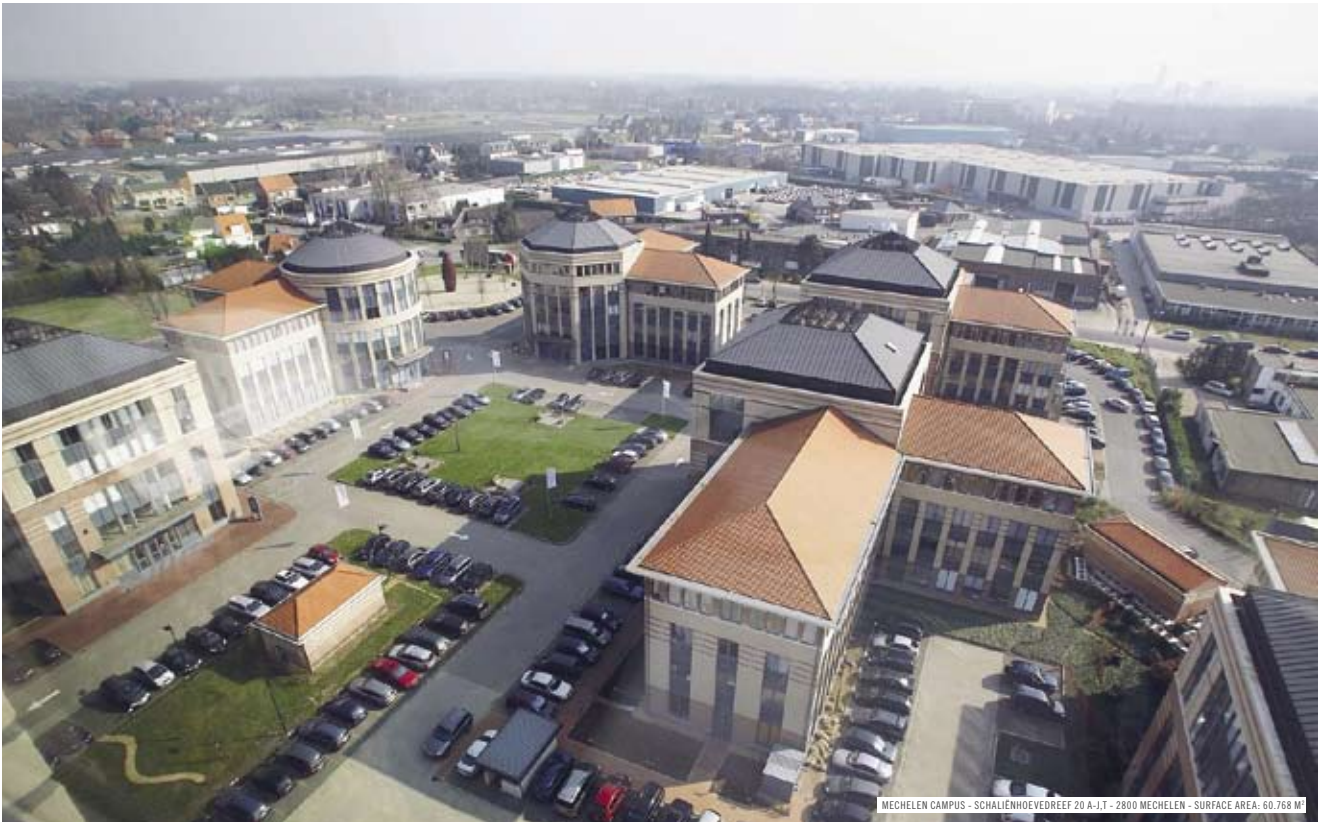
MECHELEN CAMPUS - SCHALIENHOEVEDREEF 20 A-I,T - 2800 MECHELEN - SURFACE AREA: 60.768 M 2
