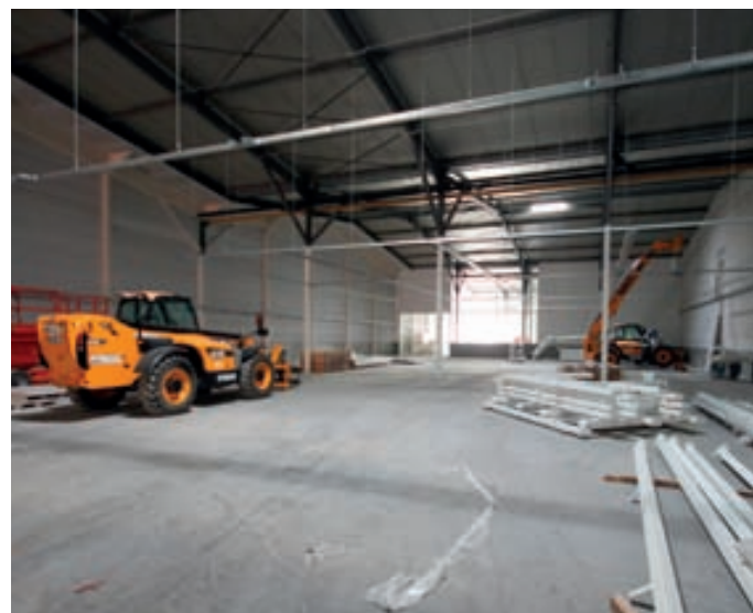
14. positioning cable ducts in workshop
