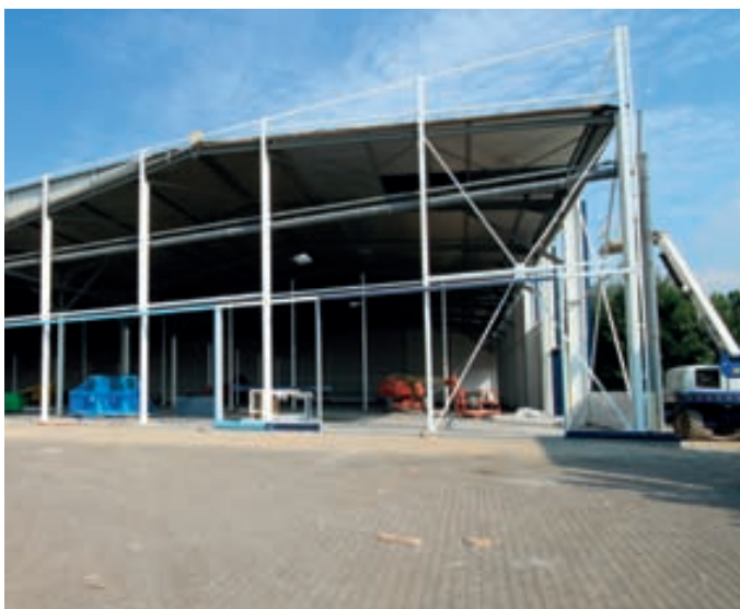
5. installation support structure for new facade cladding
