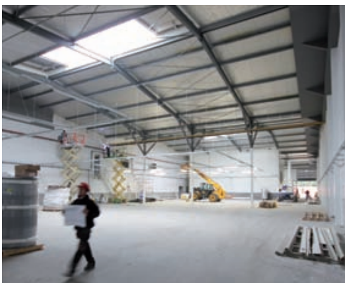
15. installation of lighting system and exhaust extraction system in workshop
