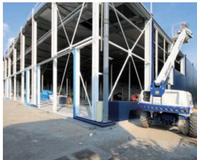
6. placing of sandwich panels new facade
