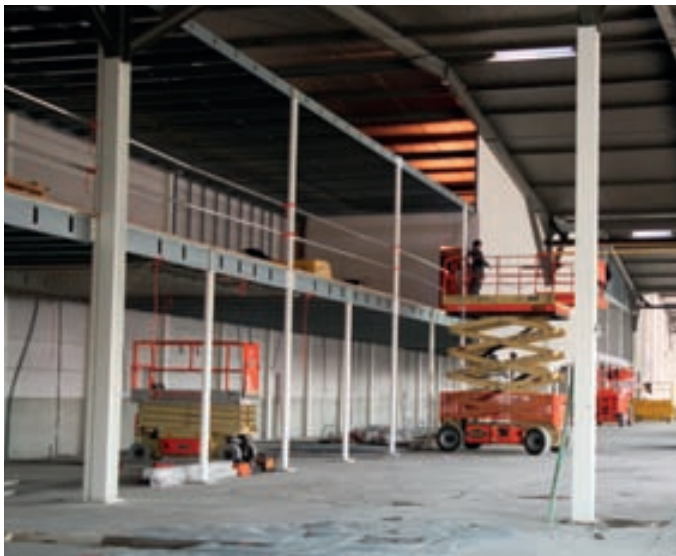
9. installation support structure for first floor offices
