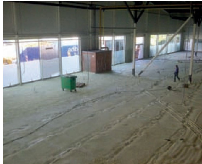
10. spraying of floor insulation in showroom
