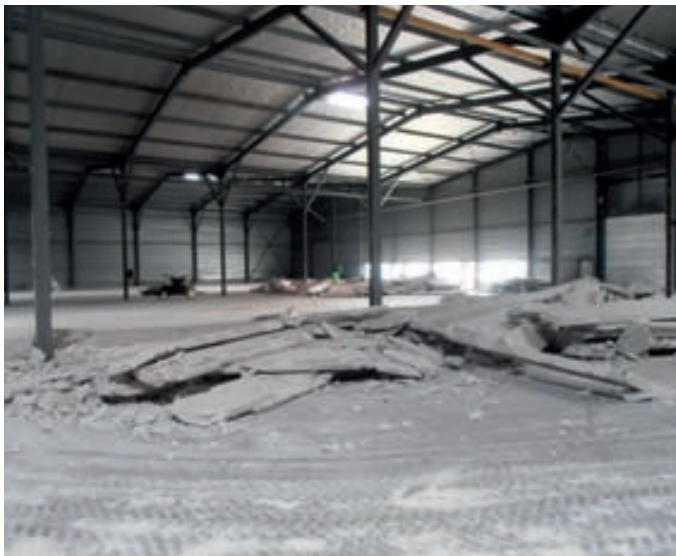
1. demolishing of existing walls
