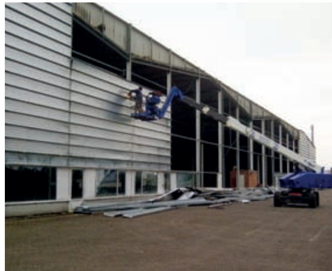
2. removal existing facade cladding
