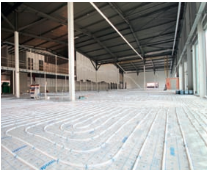
11. installation under floor heating system in showroom
