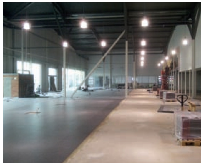
12. placement floor tiles in showroom - finishing offices
