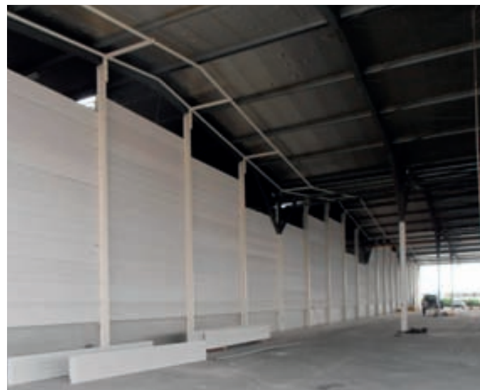
4. construction of flashover security element
