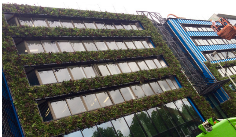
▲ Greenhouse Antwerp - Installation façade verticale
